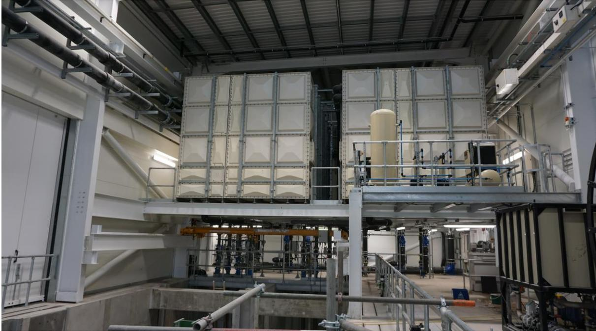
Two Header Tank Systems supplying the Testing Tank – Flows up to 200 l/s
